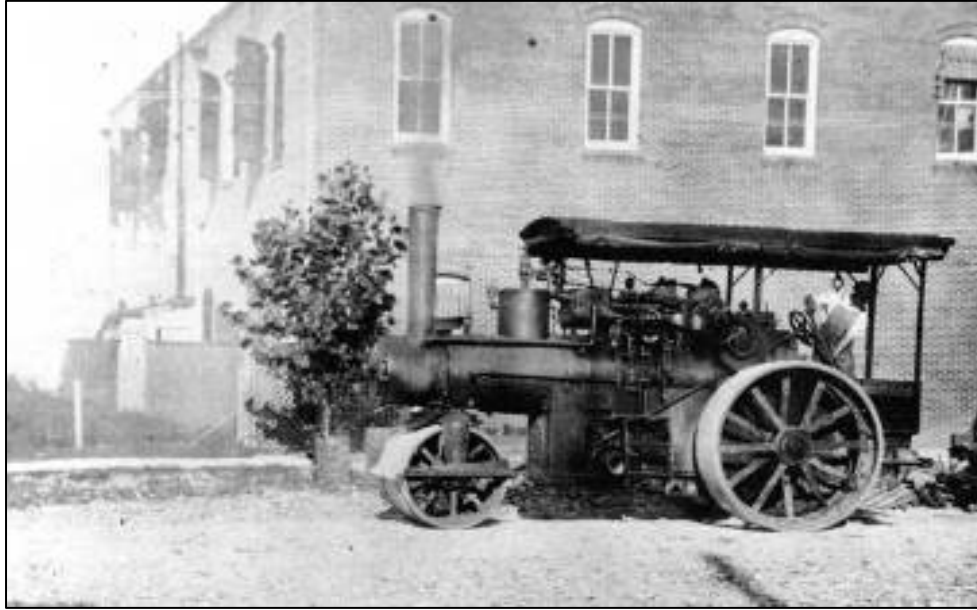
Figure 8. Steam roller, packing shells for Apalachicola roadbed in 1910. Courtesy of the Florida Memory Collection.
